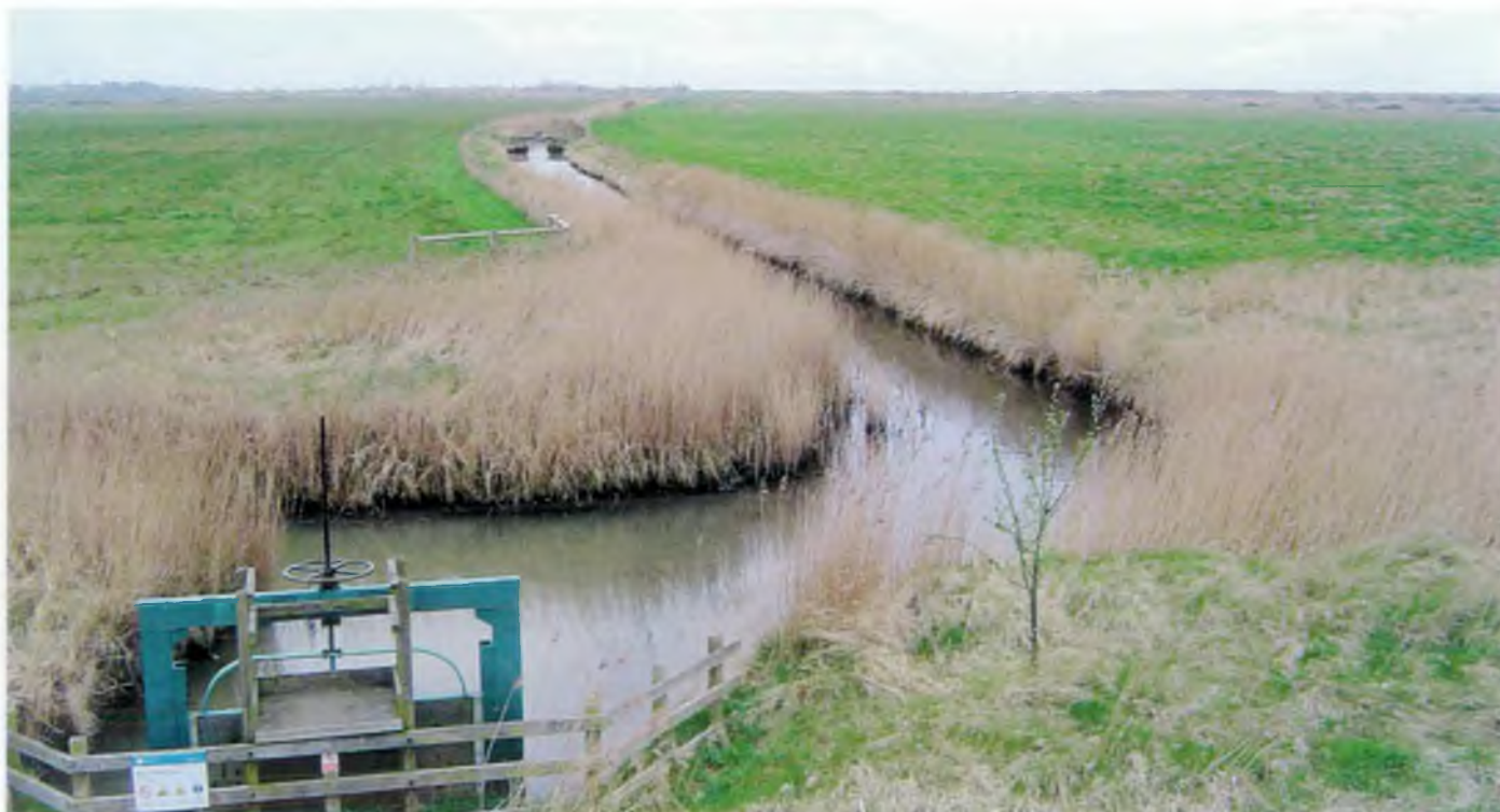
River Mun Outfall Sluice
