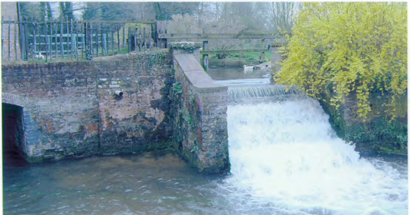
Letheringsett Mill on the River Glaven
