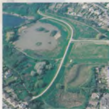
The raised dam crest
