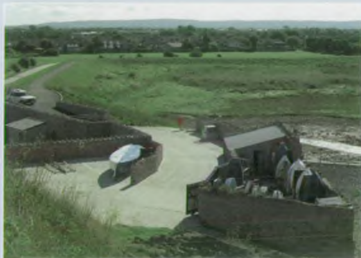
Local limestone was used to match existing boat store
