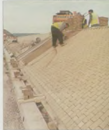
200,000 blocks were used to pave the rear slope
