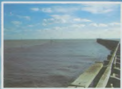
The shipping channel and breakwater at Littlehampton harbour
