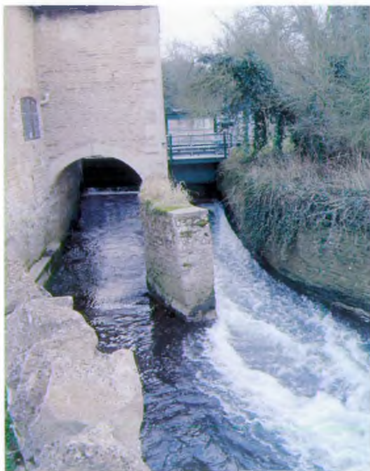
Duddington Mill Sluice
