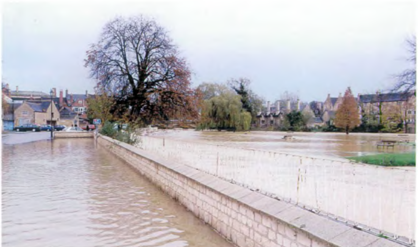
Flooding in Stamford, November 2000
