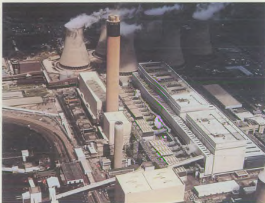
Drax power station on the Lower Ouse
