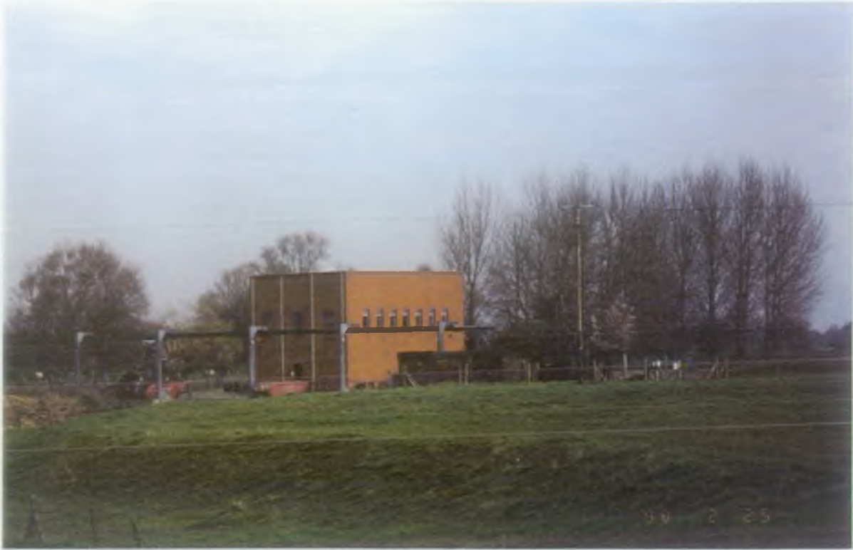
Figure. 2b : Peakirk Pumping Station
