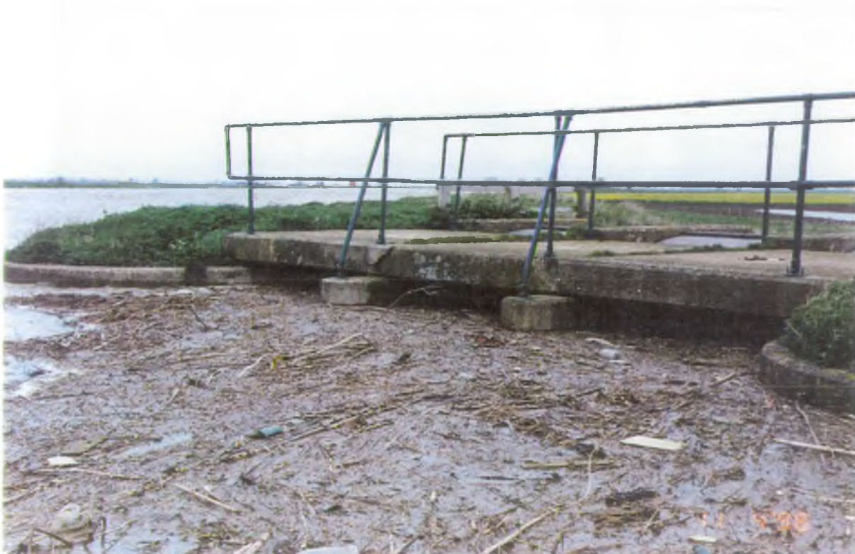
Figure. 8c : Newborough Syphon During The Easter Flood, 11/04/98
