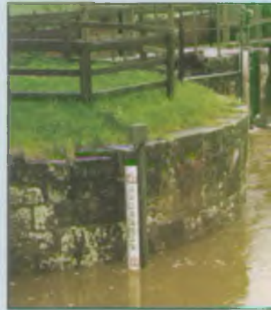
Weir Head sluice
