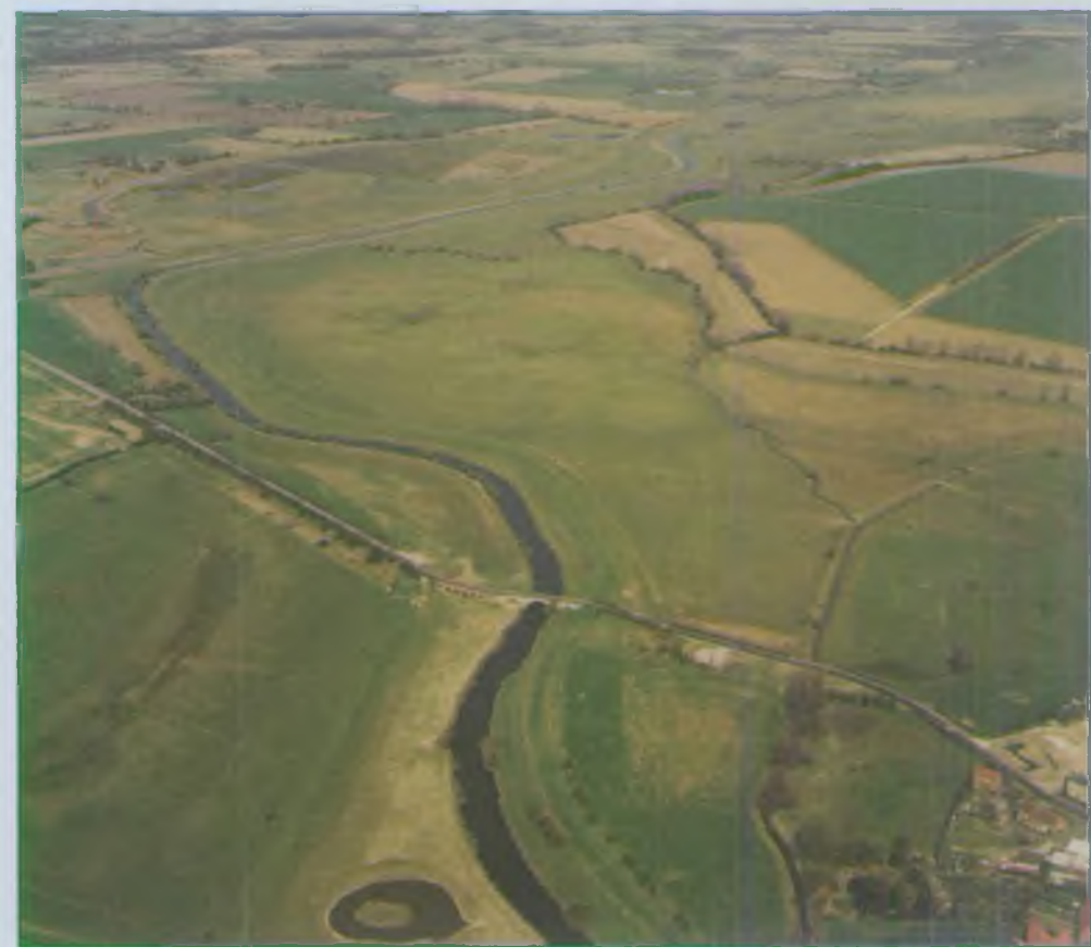
Derwent Bridge, Bubwith
