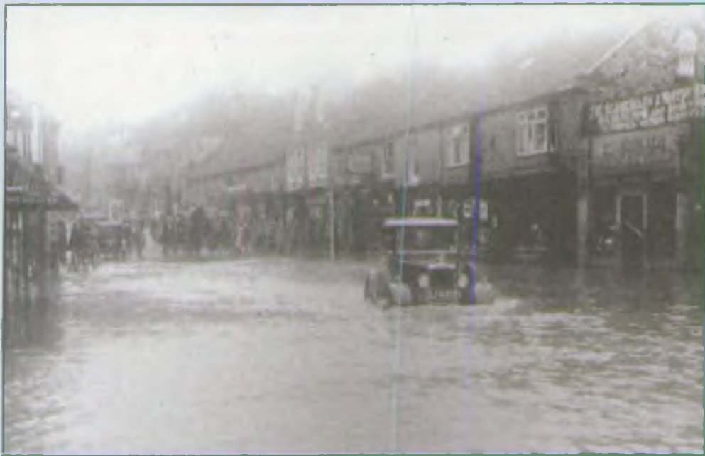
Flooded market place in Pickering, c 1930
