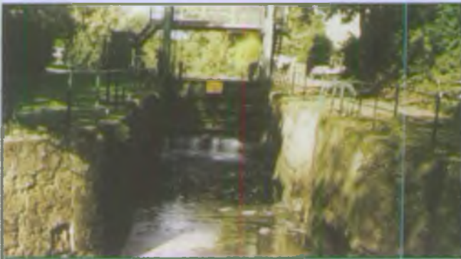
Stamford Bridge sluice
