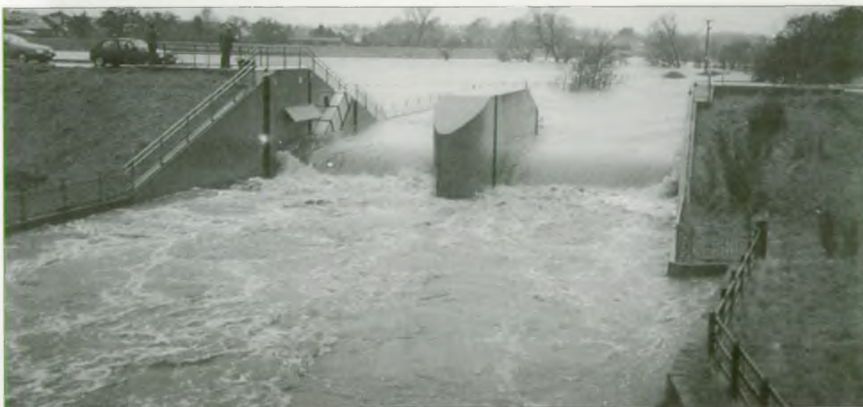
Garstang Flood Basin in operation.
