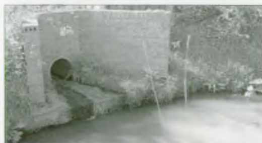
Hillylaid Pool "contaminated surface water outfall".
