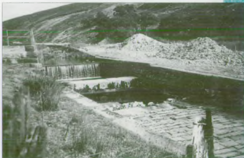
NWW intake at River Calder.
