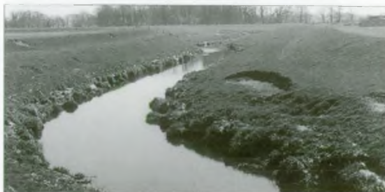
River Wyre. Treeless banks, erosion and degraded habitat.
