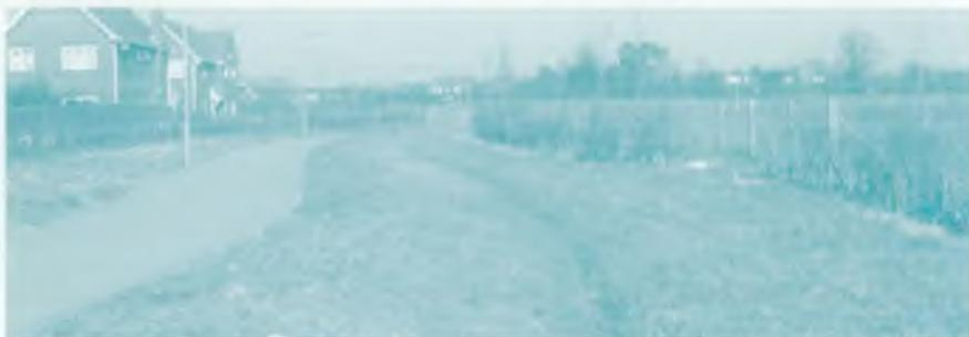
**Attenuation:** Store water at the ground surface temporarily or permanently. Balancing pond at Cherque Farm, Gosport.
