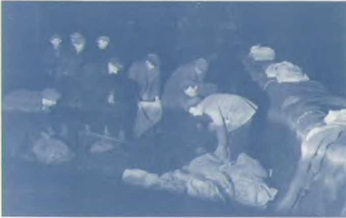
Top: Structures could not cope with the amount of water
