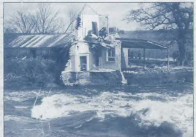
Destruction - a house is demolished by floodwater
