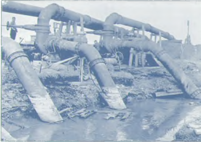
Above: Huge pumps sucked away the floodwaters reclaiming the drowned fields
