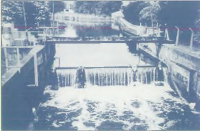
Top: New channels and cuts were dug to better handle flows
