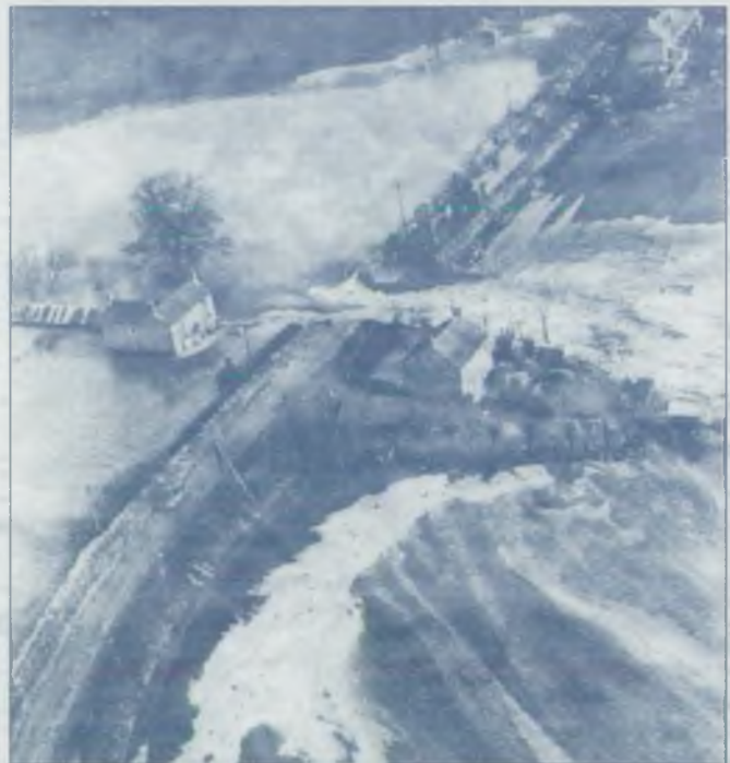
Waves of water (foreground) smash against the remaining defences
