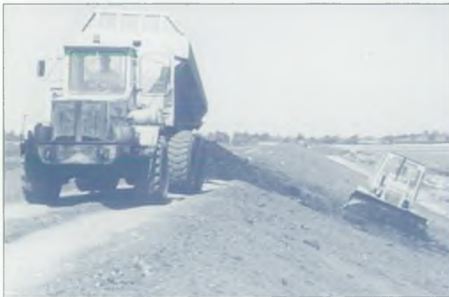
Below: Huge construction projects help to strengthen flood barrier banks
