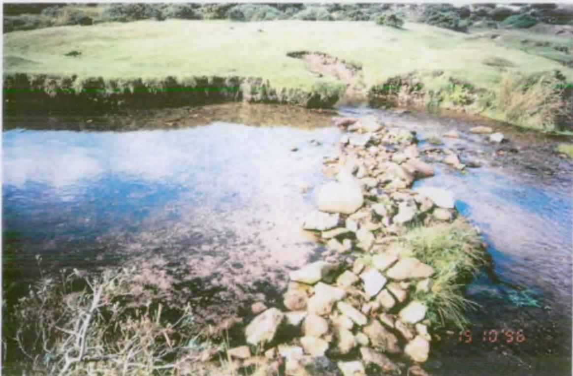
Photo (4). Dam 1, after it had been breached. Note the lack of detritus and diatom growth, removed by the increased flow rate.
