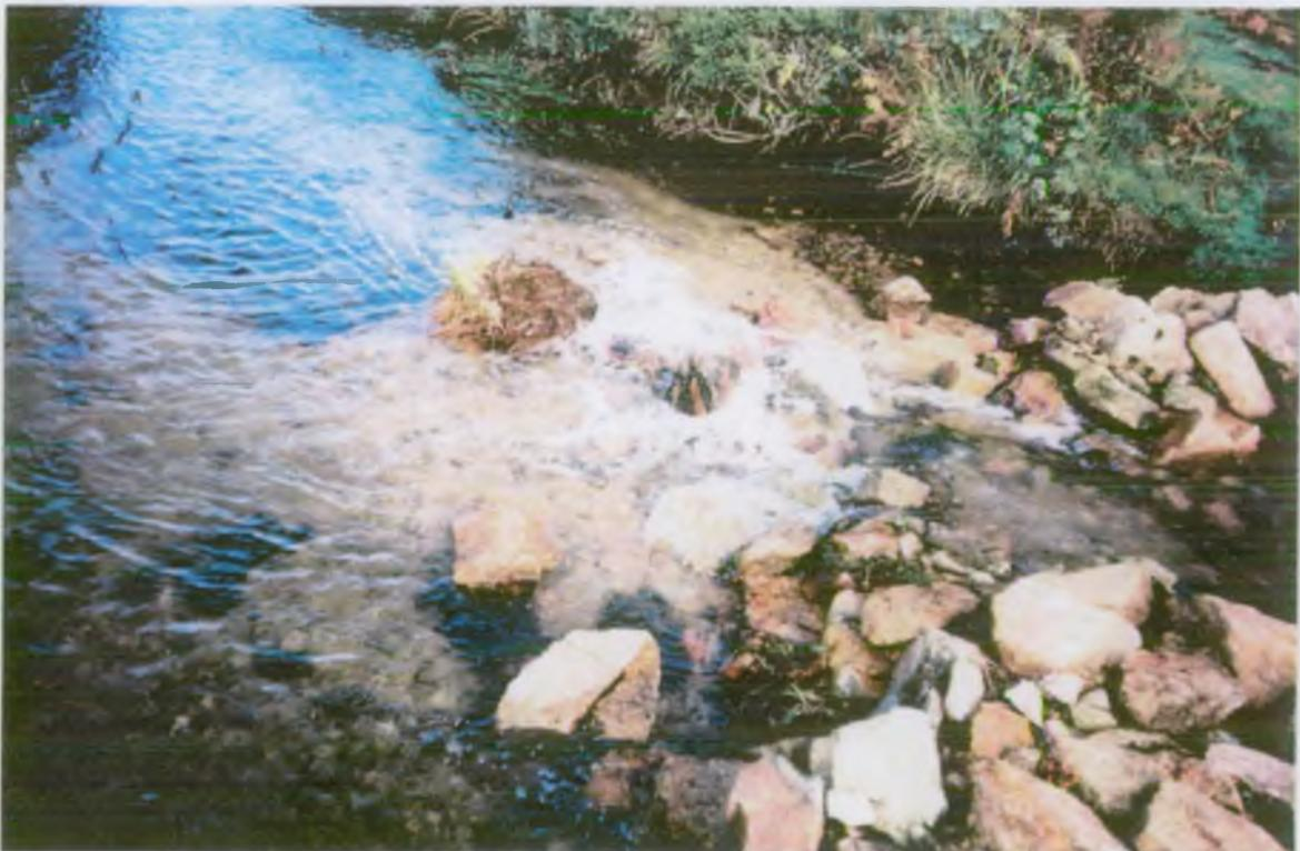
**Photo (8). Dam 3, after breaching. Note the size of turf used in construction.**
