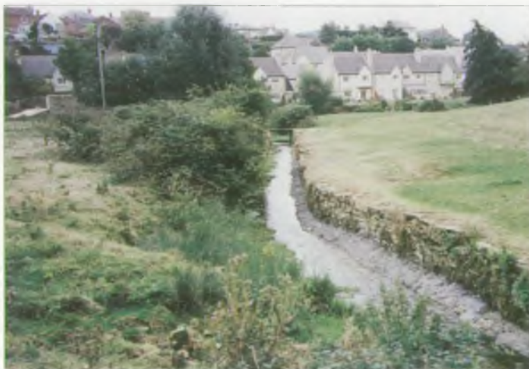
Daniels Well leat after sealing with sand bags and clay
