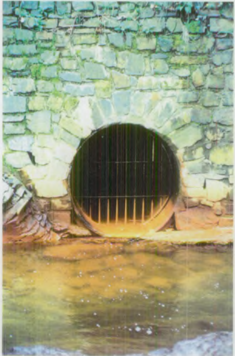
Iron hydroxide deposits in the drainage adit from Meldon Quarry and in the West Okement River downstream of the drainage adit
