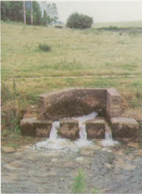
Stream support pumping, Luckington
