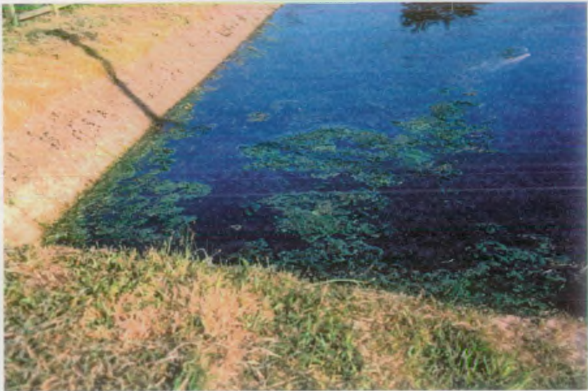
FIGURE 4. DENSE GROWTH OF ALGAE IN SILT TRAP
