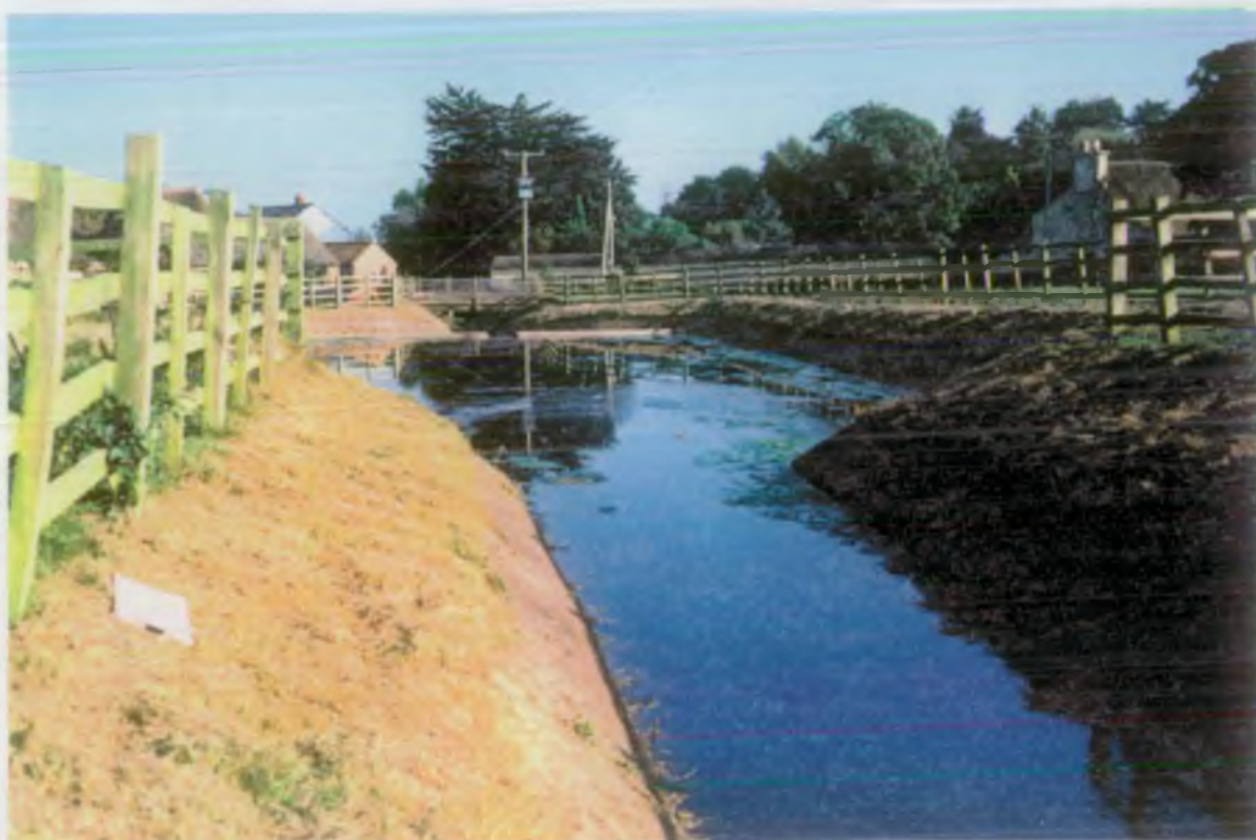
FIGURE 2. GENERAL VIEW OF SILT TRAP
