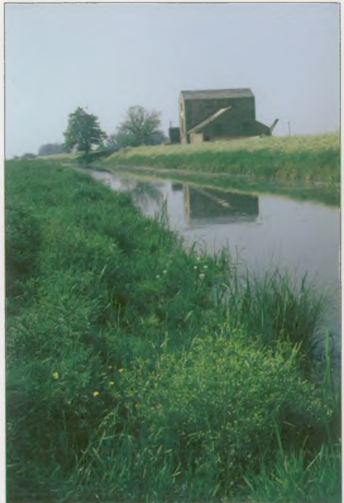
Counter Drain, Bedfordshire
