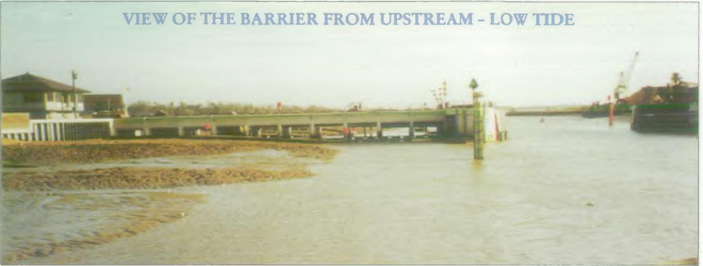
Barrier, the Colne Barrier is designed to resist the highest tide likely to occur once in a thousand years. The barrier gates are normally open so that river traffic and the ebb and flow of the tide will continue, and will only be closed when a high surge tide is forecast.
