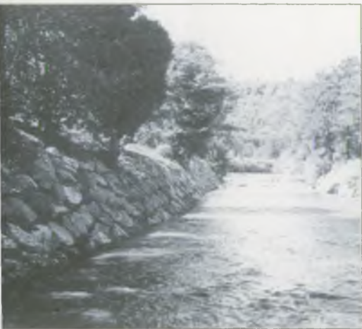
Flood defence works at Cwmilas
