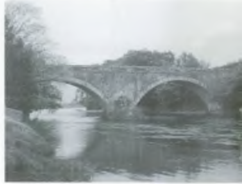
Ouse Bridge, Bassenthwaite
