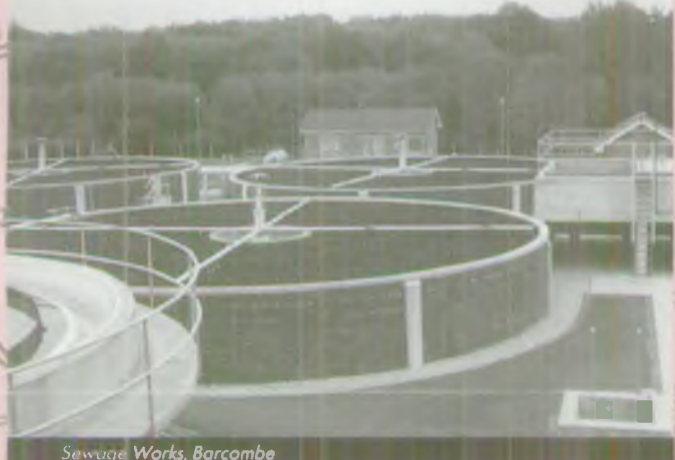
Sewage Works, Barcombe
