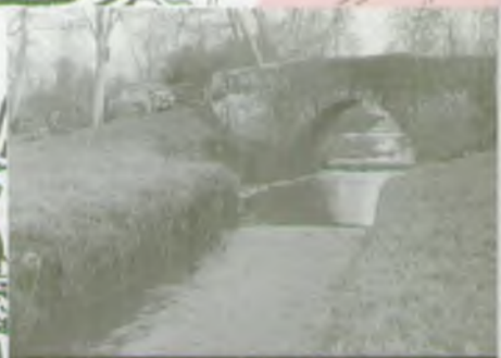
Fish Ladder, Barcombe Mills
