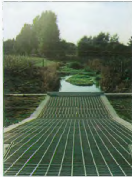
Bear Brook flume view looking downstream
