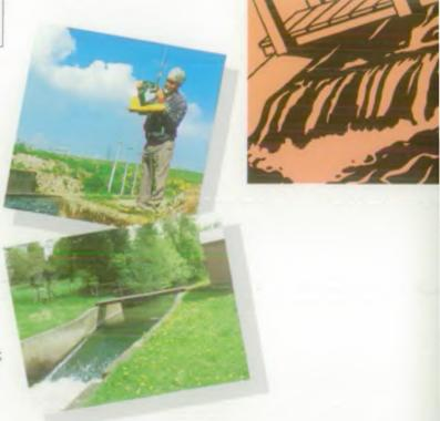
At gauging stations, because the processes of erosion and deposition continually change the shape of natural rivers, it is sometimes necessary to build stable structures such as weirs. A calculation is then used to convert the level of the river accurately into flow.
