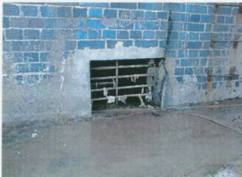
Storm discharge overflow in outfall chamber
