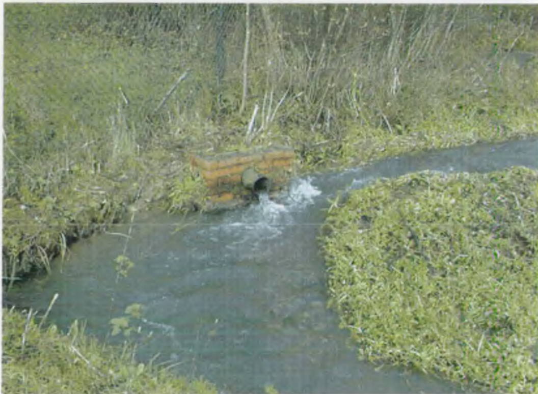
Final Effluent Discharge Situated Downstream From Storm Discharge.
