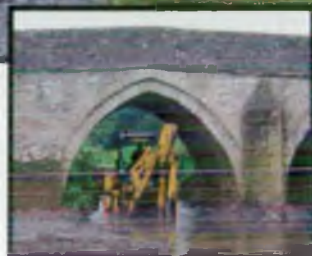
Before, during and after the removal of 128 tonnes of silt at Tunbridge
