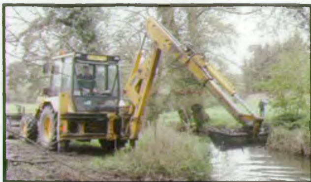
Dredging the millstream
