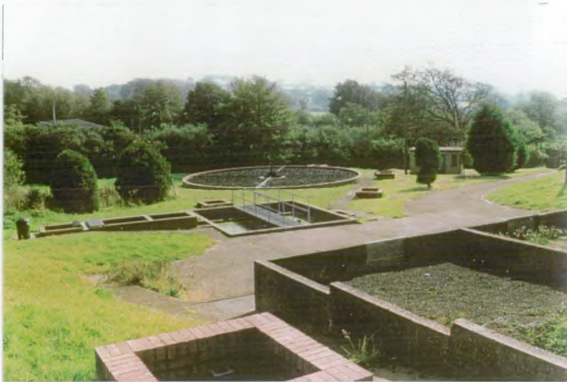
Photograph 1. Bradworthy S.T.W. showing screening tank and biological filter bed.
