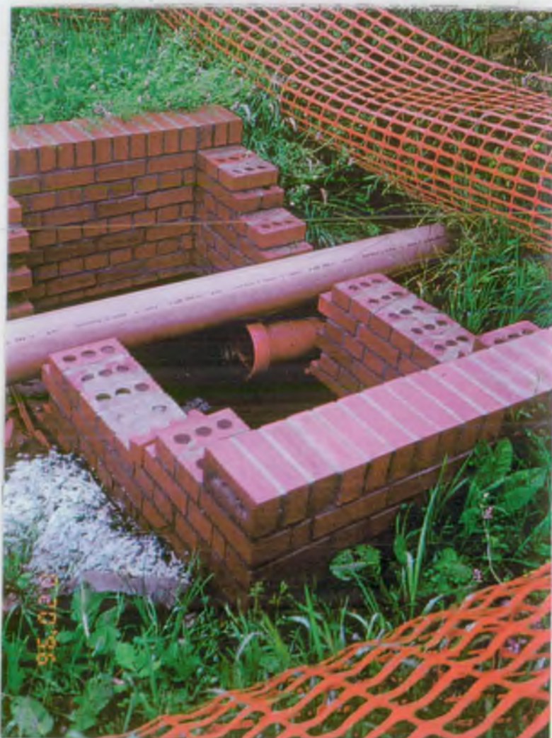
Photograph 4. Storm overflow inspection chamber. containing two pipes while under construction
