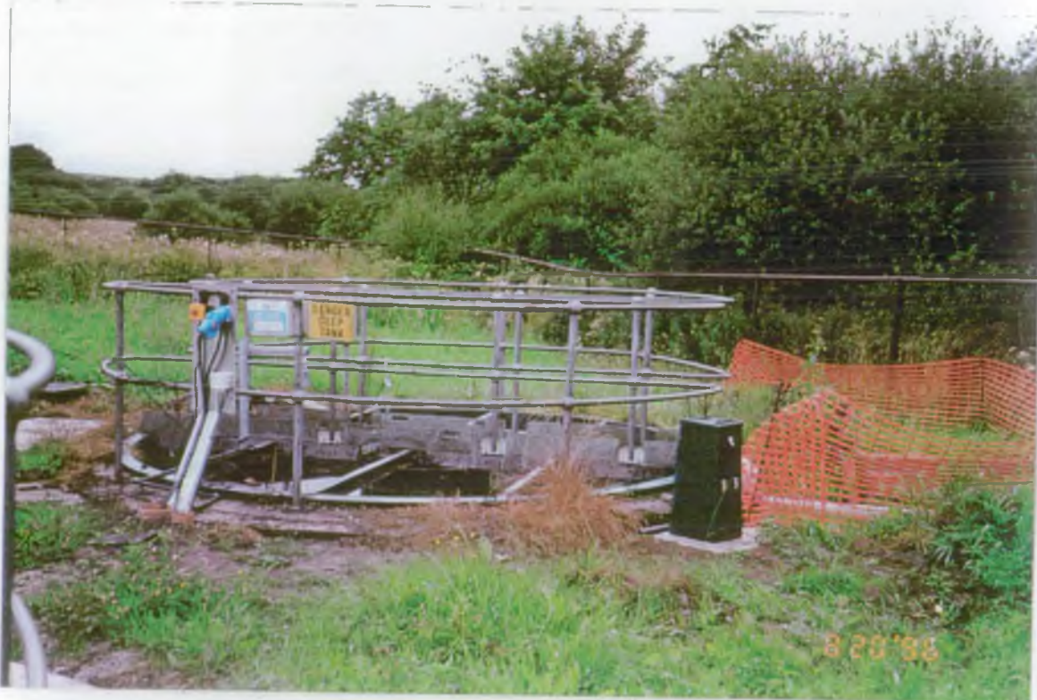
Photograph 4. Storm overflow inspection chamber. containing two pipes while under construction
