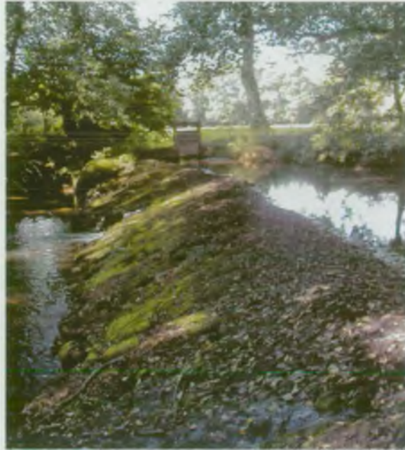
Showing very low flow conditions. No flow over top of weir.
