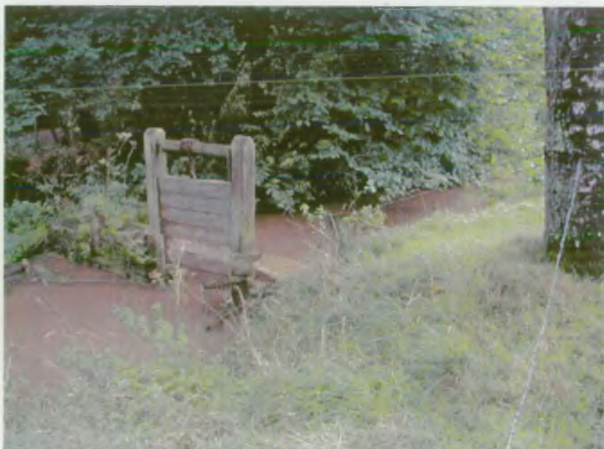
Mill Leat entrance from River Dalch Side of Weir.
