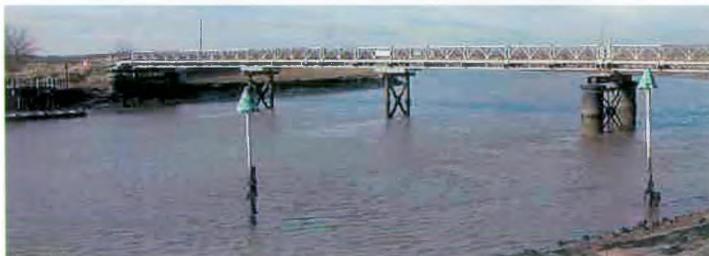
Bailey Bridge, River Blyth
