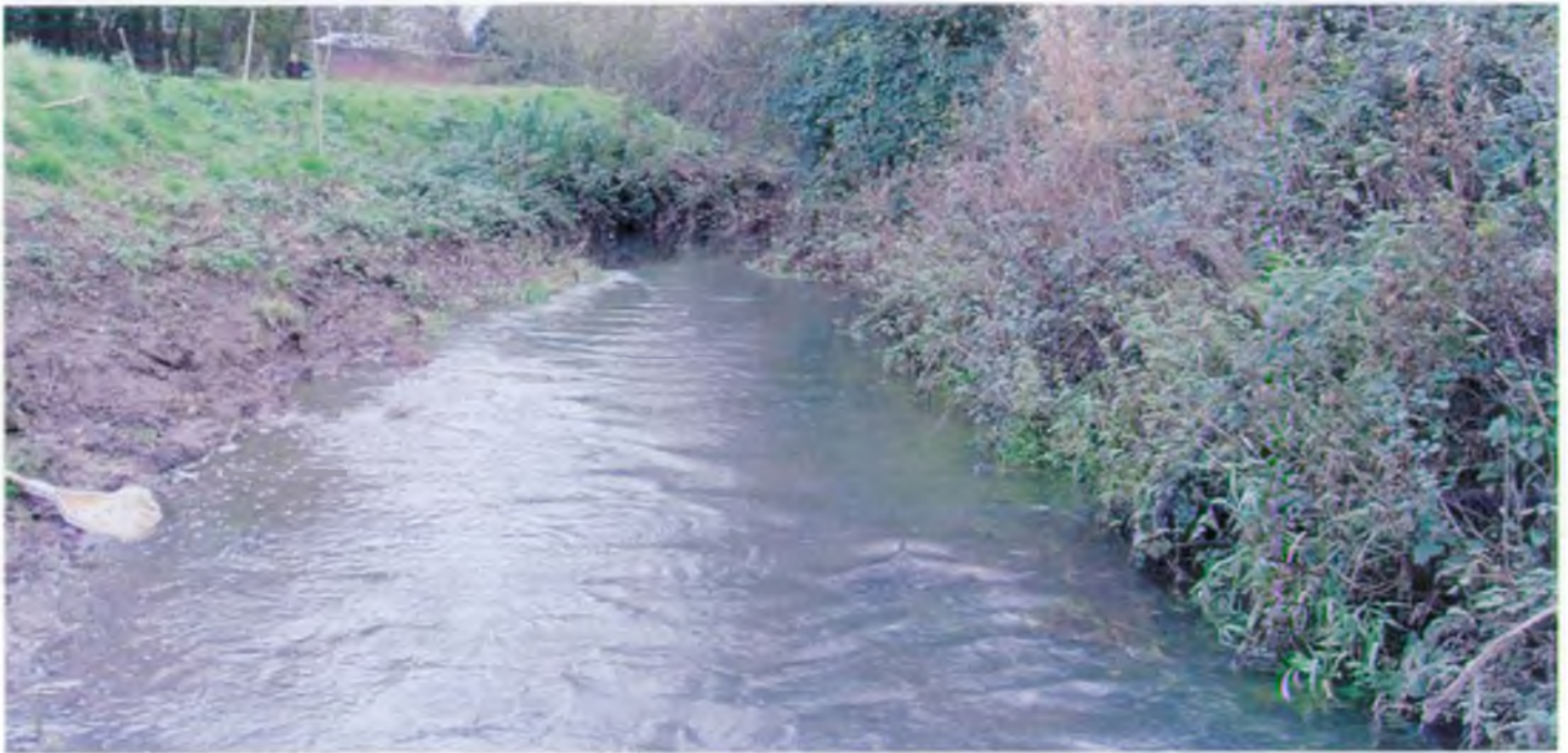
Farnham Bridge, River Alde
