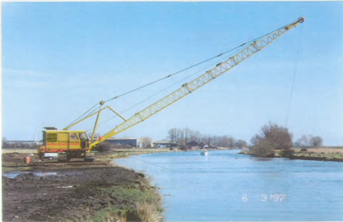
Figure 2.2: Dredging Work on the Ely Ouse at Ely
