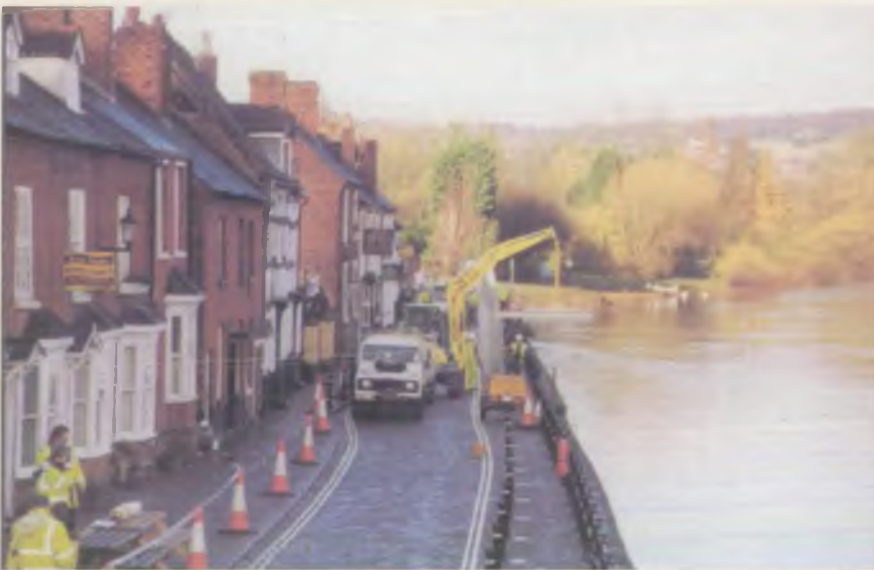
Bewdley - erecting the defences
