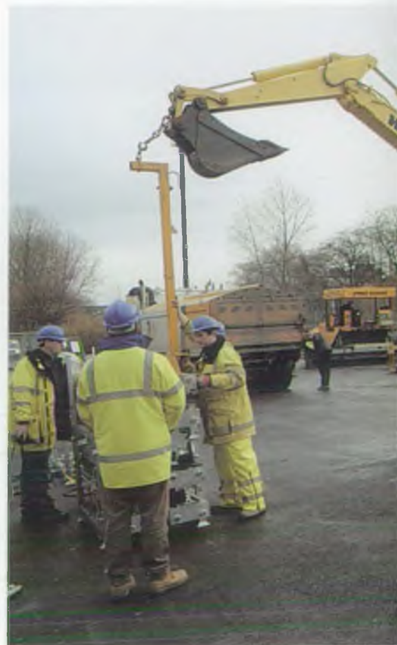
River Severn, Frankwell, Shrewsbury, September 2002
