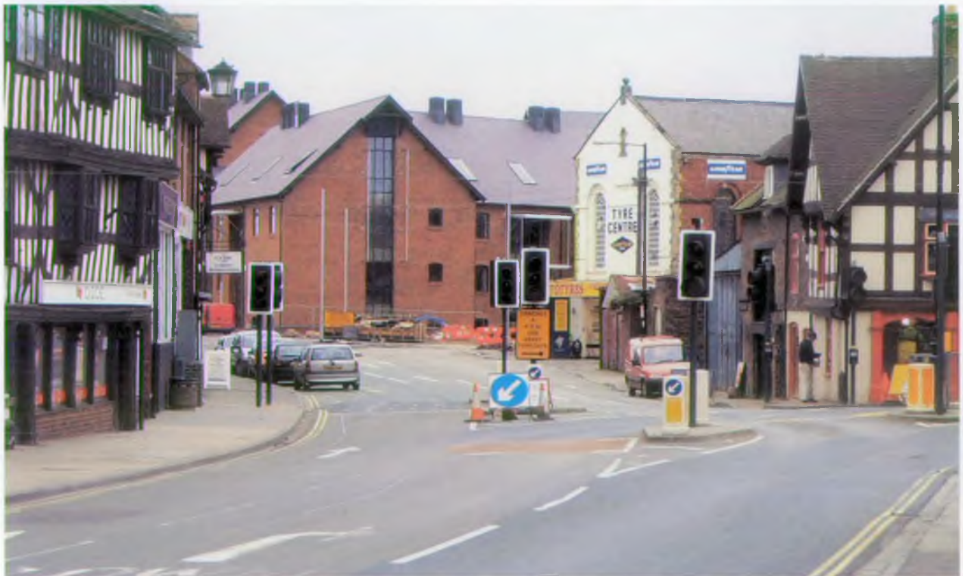
February 2004 flood © Shropshire Star
