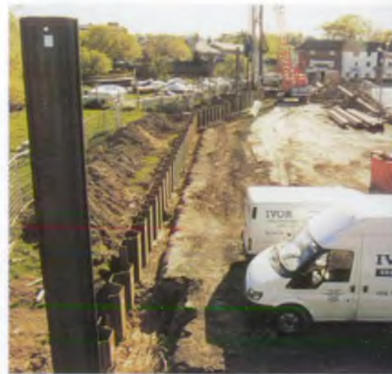
Building the flood defences, Frankwell, April 2002
