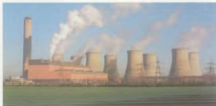
Cottam Power Station
