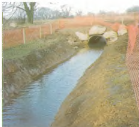
The open channel between the river and the pool
