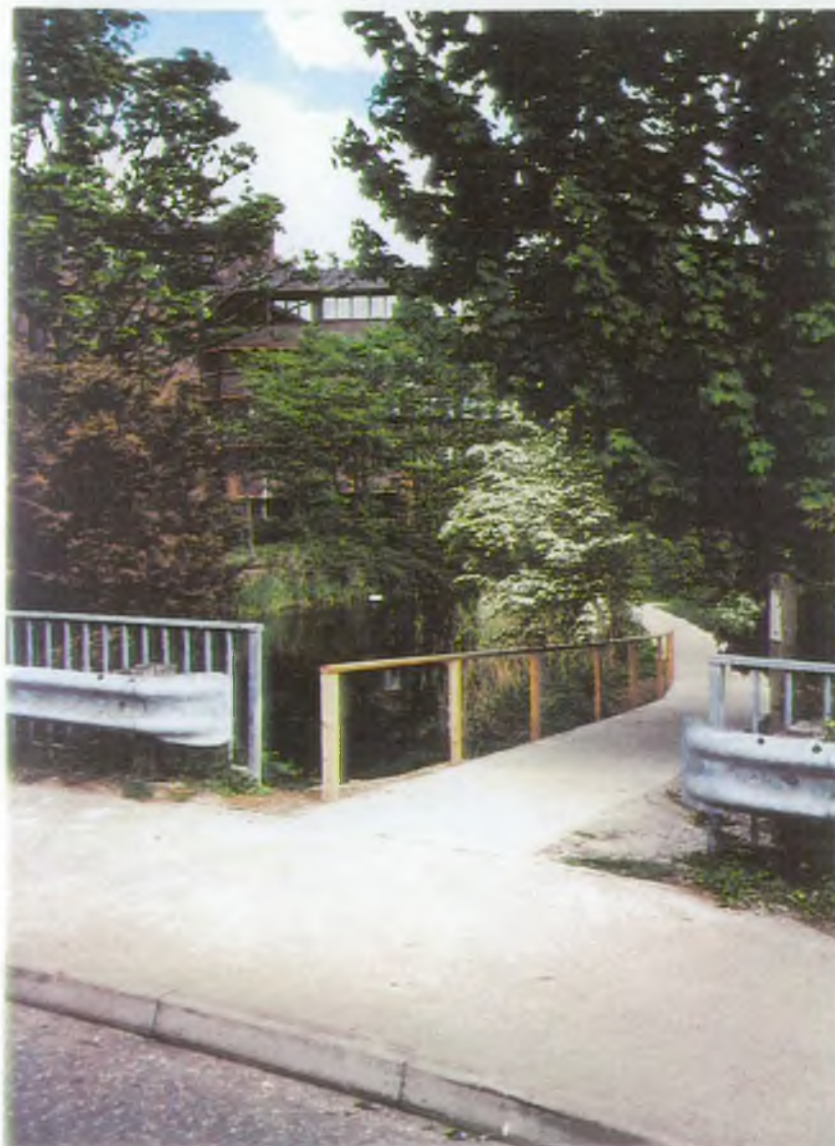
Photo 20 Alderman Canal with access ramp
