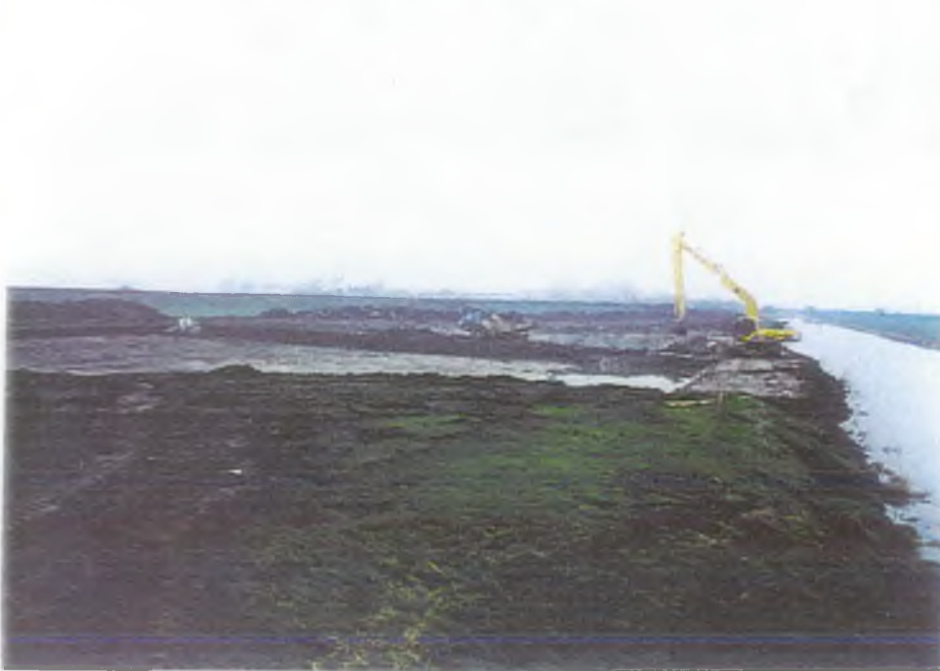
Photo 4 Work beginning on the Louth Canal fish refuge.
