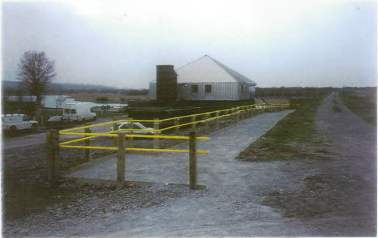
Photo 14 Humber embankment with access ramp
