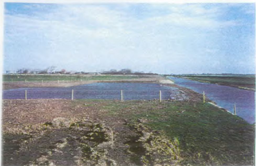
Photo 5 The completed fish refuge
