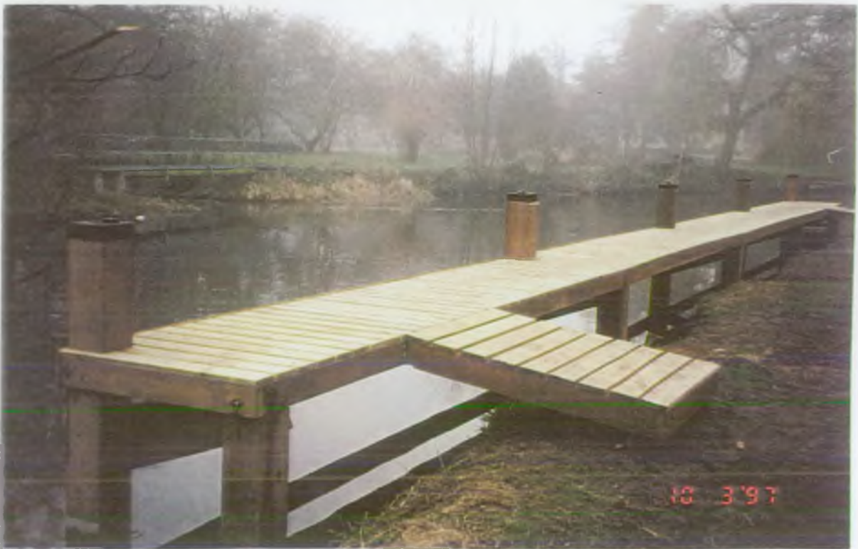
Photo 35 New landing stage in Brandon
