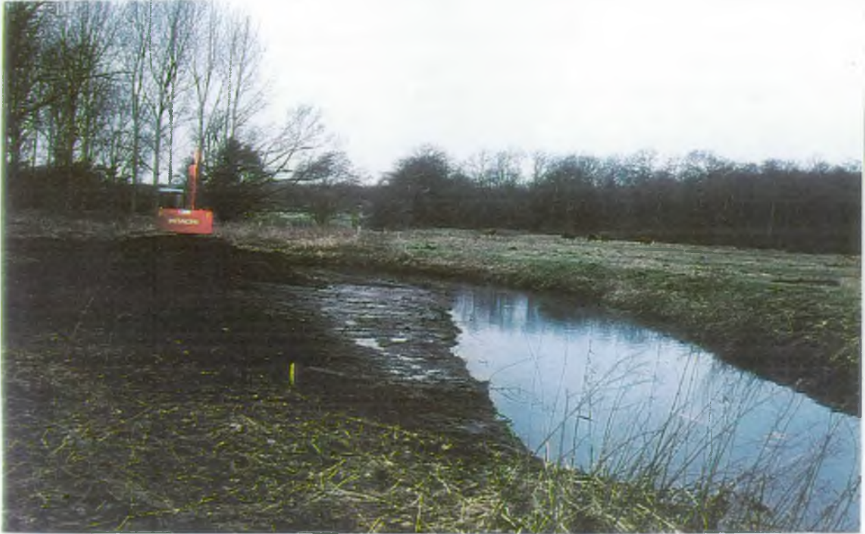
Photo 10 The completed bank reprofiling at Hoe Rough.
