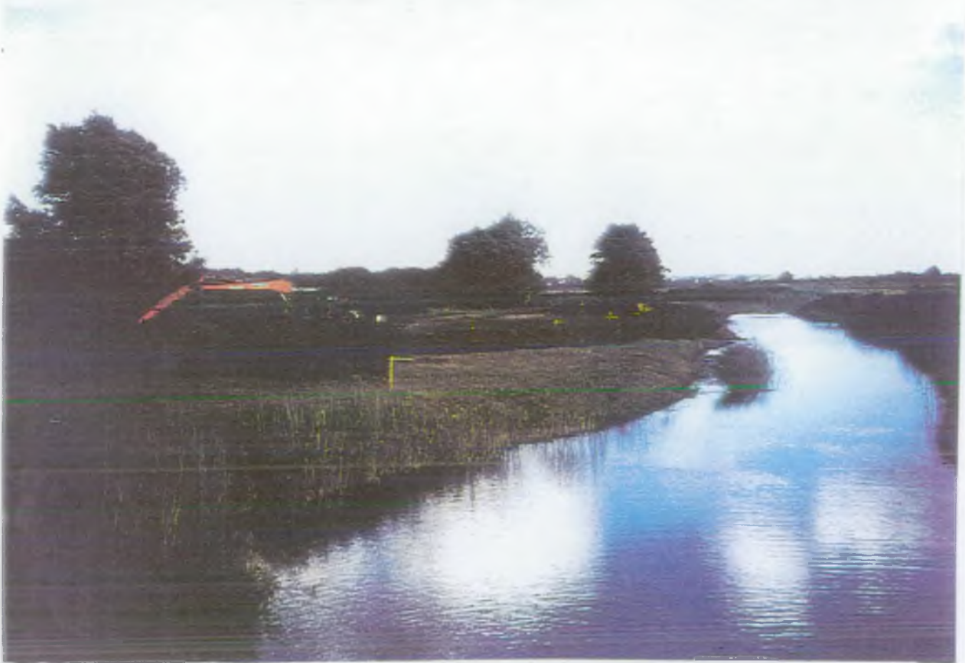
Photo 30 Spoil being removed to create reedbed
