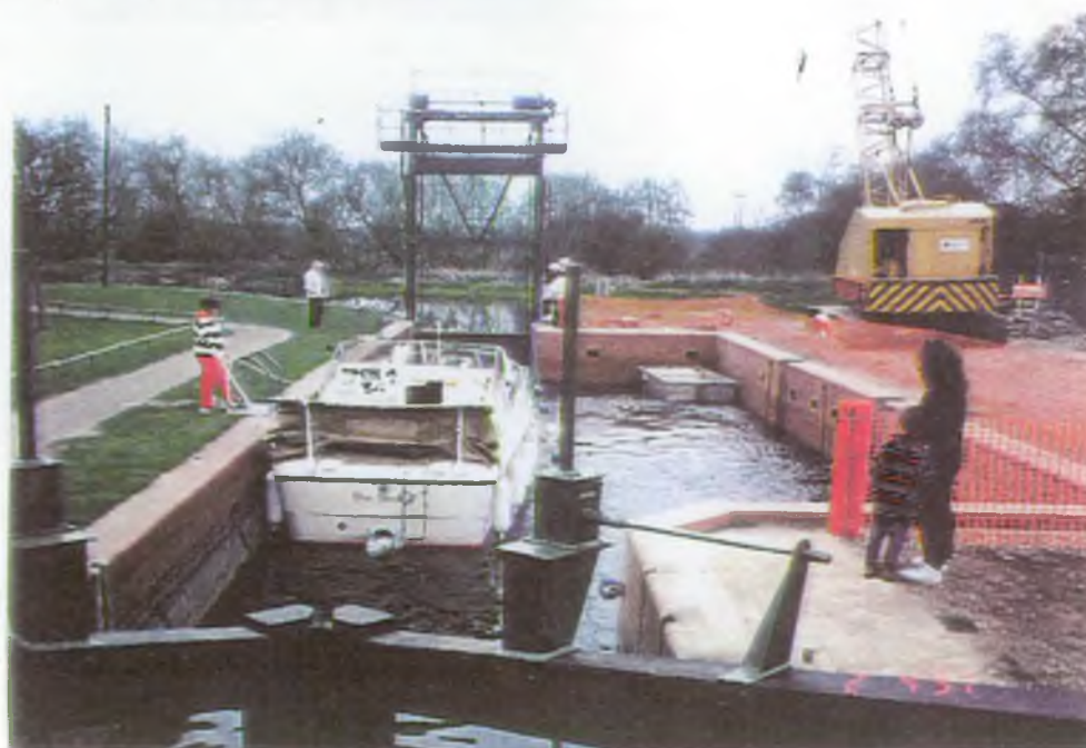
Photo 37 Boat using newly completed lock
