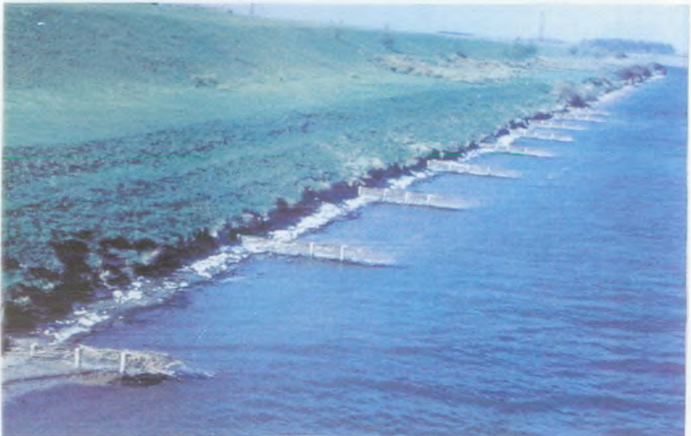
Photo 2 The willow croys installed on the Relief Channel - Jan 97
