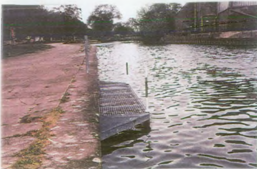
Photo 15 Canoe launch site at Wellingsborough embankment
