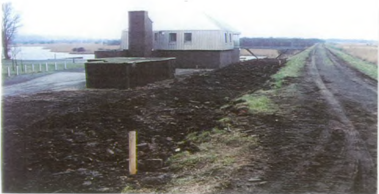
Photo 13 Humber embankment before ramp constructed
