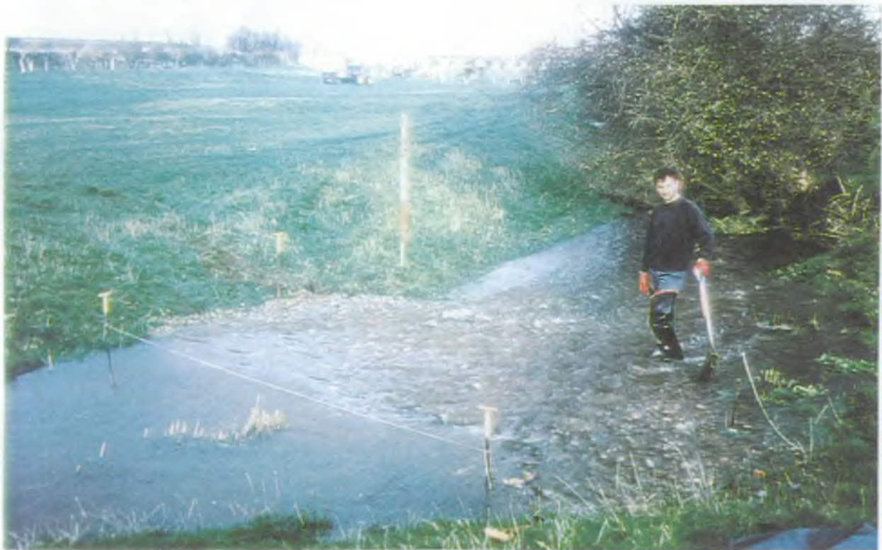
Photo 8 Created riffle on the Binham Tributary
