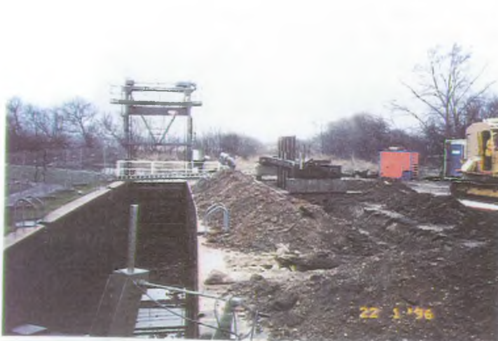
Photo 36 Lock widening of Eaton Socon lock
