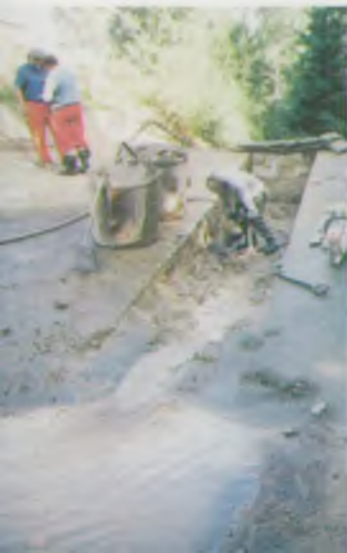
Denil Fish Pass under construction
