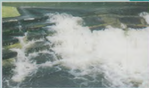
Hurn Weir after construction
