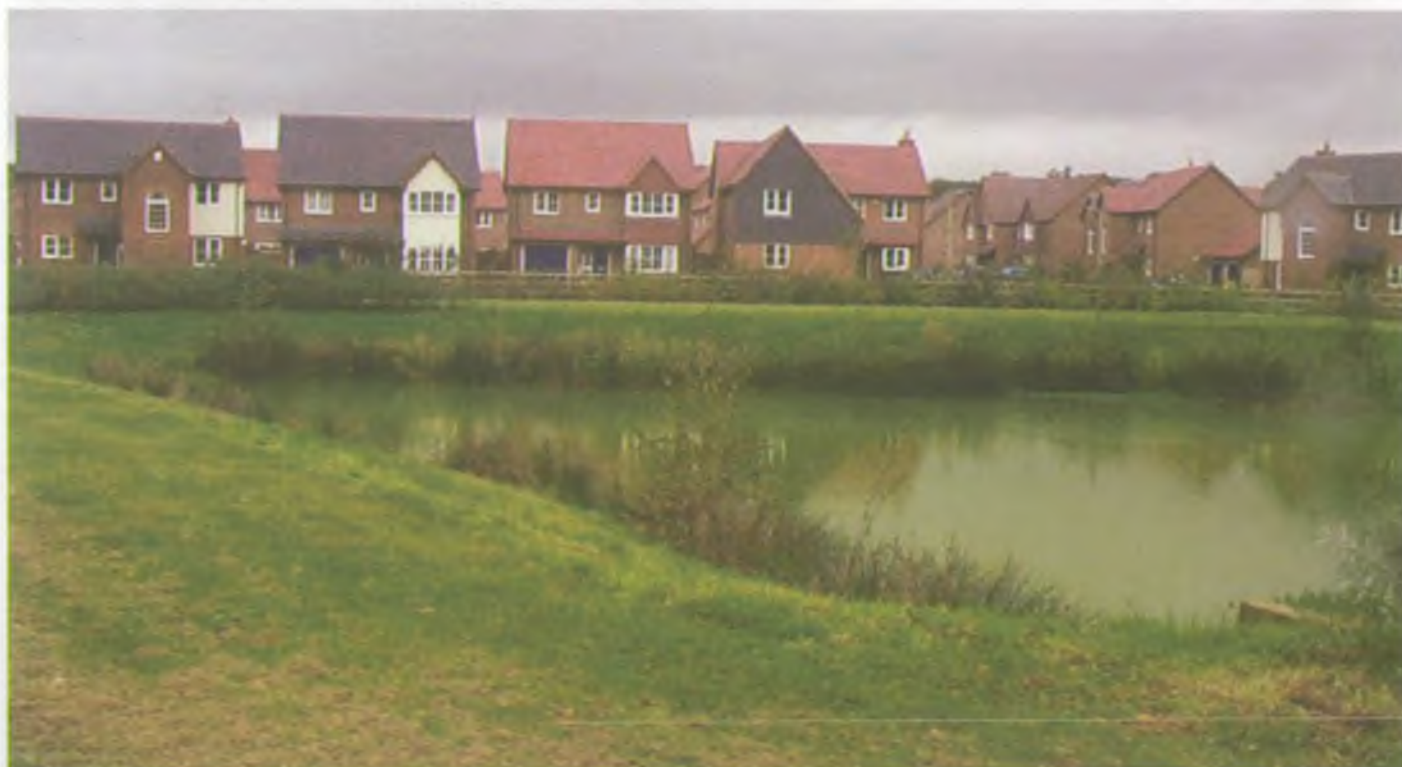
Knightwood surface water balancing pond in Chandlers Ford – a Sustainable urban Drainage scheme
