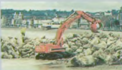
▲ Construction of rock armour groynes (Preston Beach sea defences, Weymouth)
