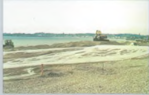
▲ Moving beach material into place (Preston beach sea defences, Weymouth)
