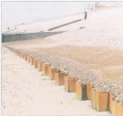
Erosion of wall, concrete worn and damaged. Fallen beach levels expose the toe of the wall
