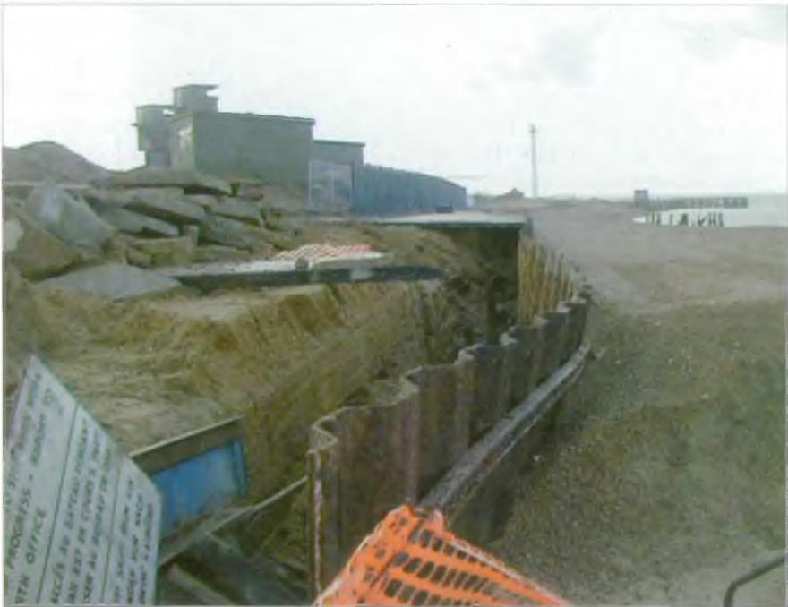
Sheet piling failure has allowed the land behind to erode
