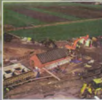
New pumping station under construction
