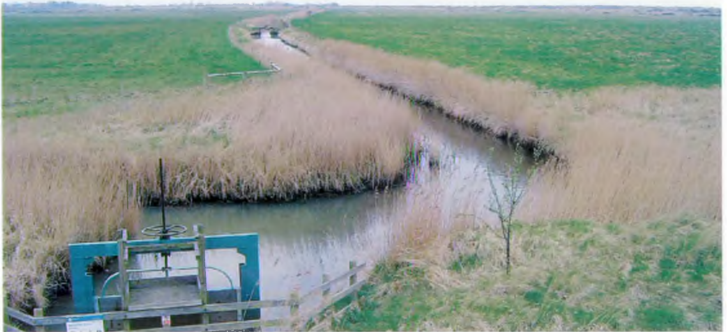
River Hun Outfall Sluice
