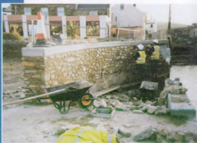
▼ Local stone was used wherever possible to build the defences
