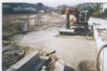
▲ The boat lake drained, enabling the culvert to be built
