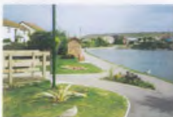
▲ The completed project - the culvert lies beneath the grass adjacent to the lake
