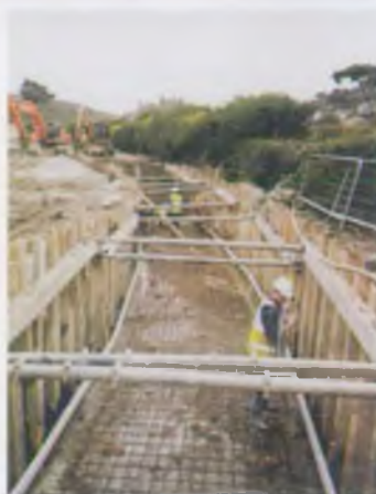
▲ The culvert under construction
