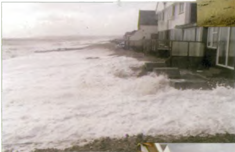
Storm conditions around Pevensey Bay
