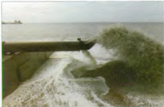
Shingle being pumped onto the shore
