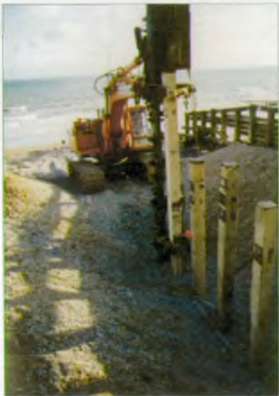
Constructing timber groynes
