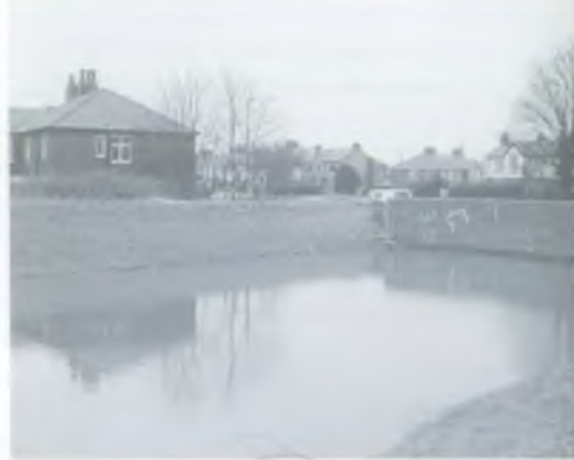
Tidal embankment, Liggard Brook. Note vulnerability of adjacent development.
