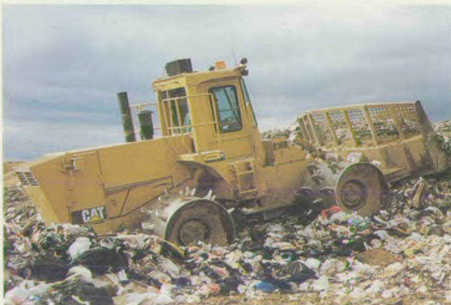
Compacting waste at a landfill site
