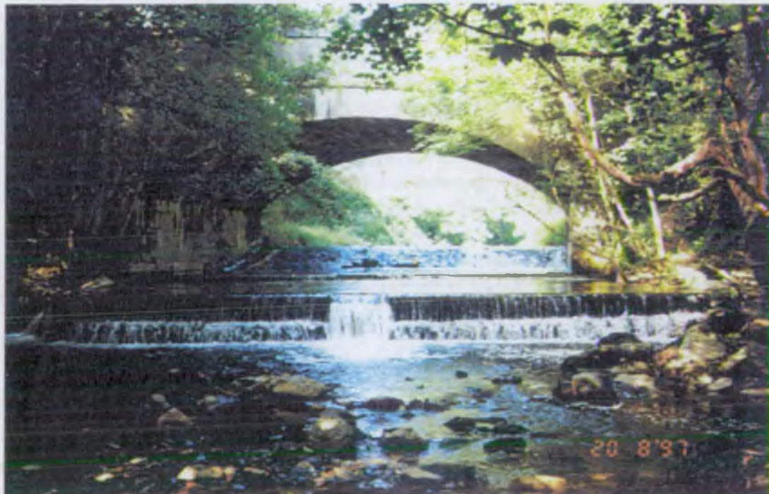
Photo 1. Yealm Bridge and weirs
