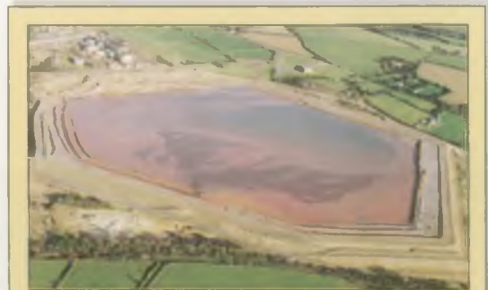
The metalliferous sediment settles into the Clemows Valley Tailings Dam which is designed to store mine tailings arising from milling operations carried out on the site.
