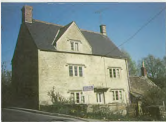
Top: Looking upstream to Doncombe Mill at Ford Middle: Derelict Undershot Wheel at Slaughterford Rag Mill Left: Ford Mill House
