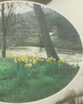
Main photo: 1982 flooding at the confluence of the By Brook with the River Avon at Bathford For left: Reel World recording studios, Box Mill Middle: The bridge at Bathford Top right: Roofs of Portals in the By Brook valley, Bathford
