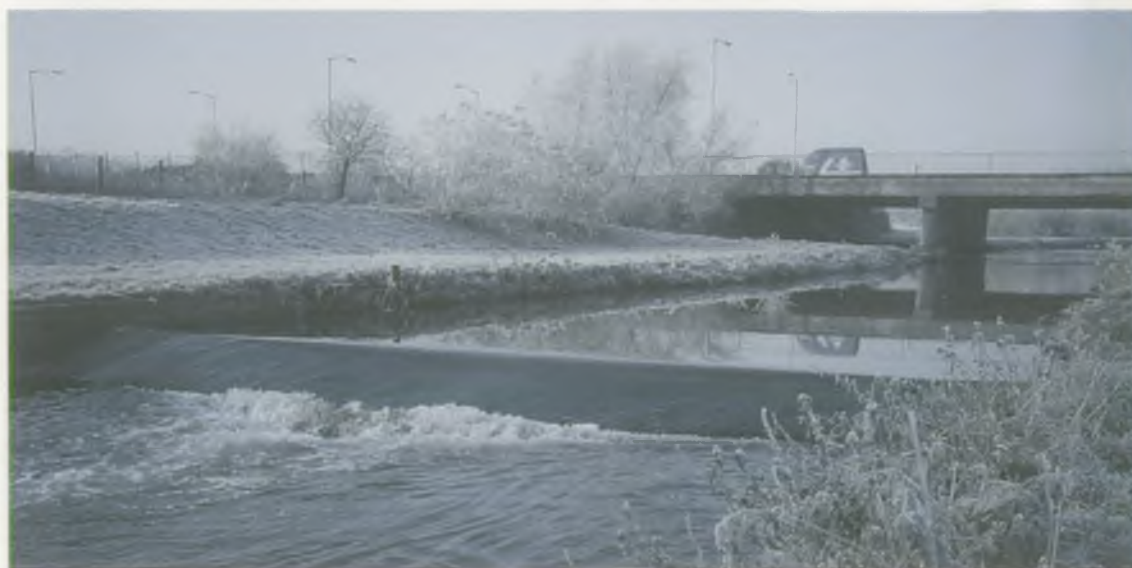
GAUGING WEIR ON THE COLE AT MOOREND AVENUE
