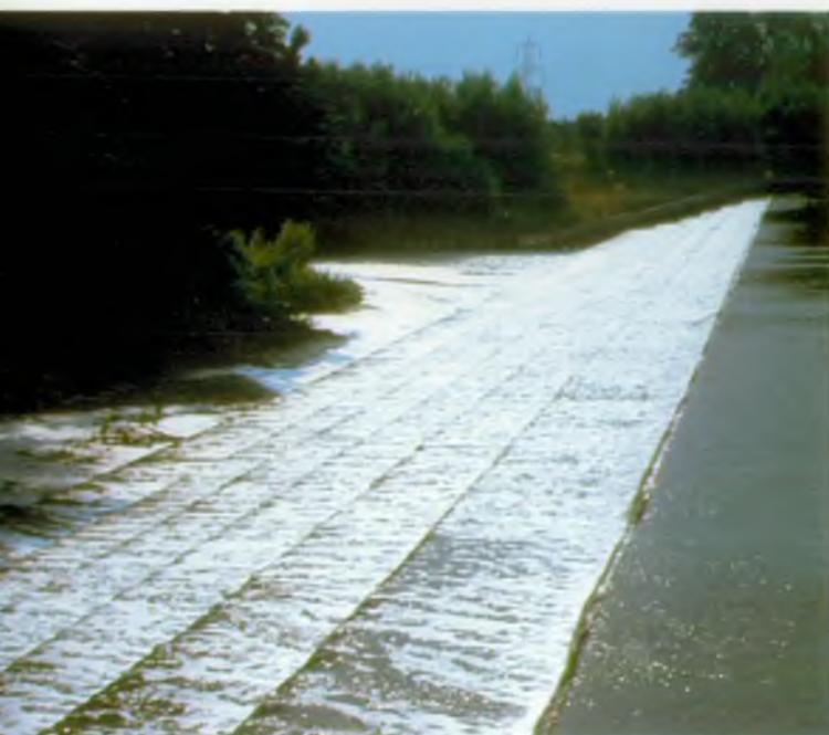
At Kegworth the “Shallow Lock” was lowered and a new “Deep Lock” was constructed to replace the existing deep lock. In the latter case, British Waterways funded and constructed the approaches to the new lock. Both the river and canal bridges were underpinned, the channel regraded between Kegworth Bridge and Kegworth Weirs and the length of the main weir was increased by 35 metres.
