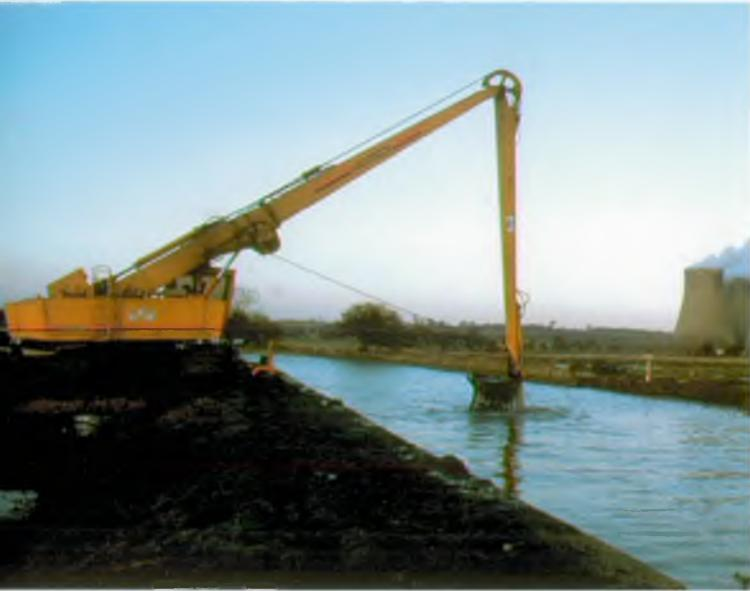
At Ratcliffe-on-Soar earth embankments approximately 1.5 metres (4.9 feet) high have been constructed alongside the village boundary to prevent the frequent flooding of the village. Landscaping including tree planting was incorporated into the scheme.
